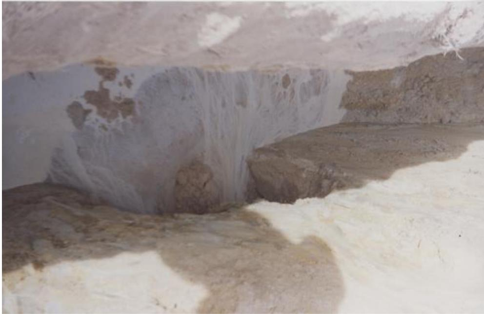
Figure 11: showing water gushing from the side wall of the trench prior to plastic insertion.
