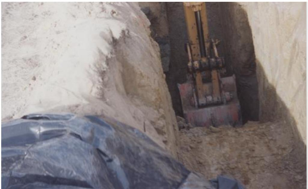
Figure 10: Showing trench being prepared to insert the plastic liner.
