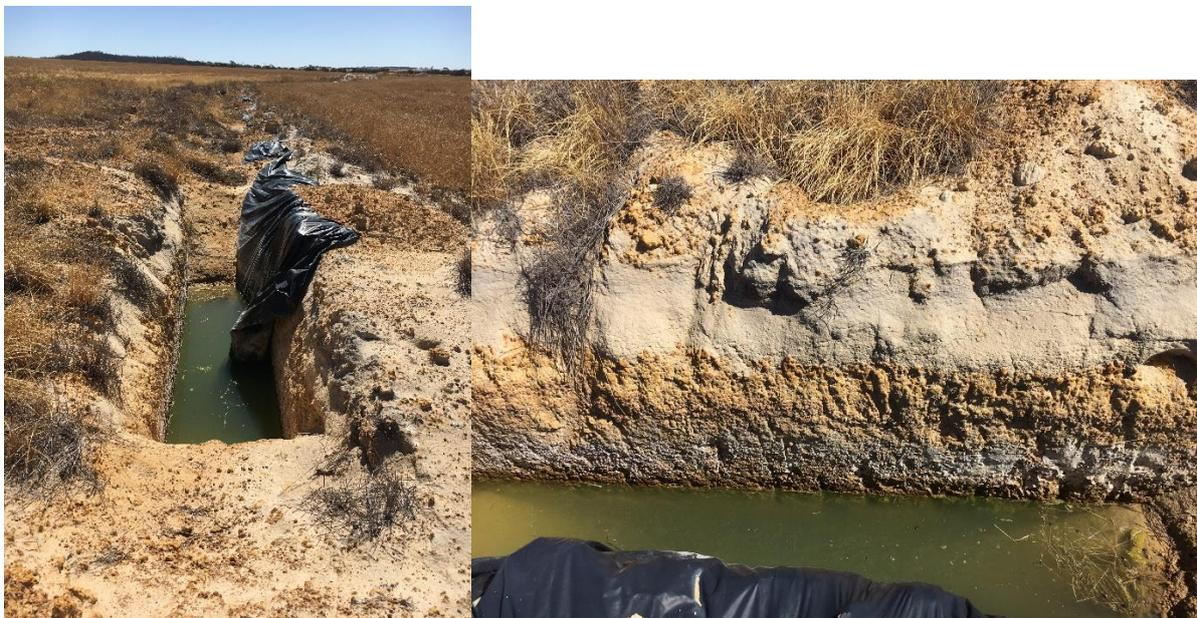
Figure 6: This image shows barriers being installed, water can be seen perched above the C horizon (approx. 1.6m) has seeped into the trench.
